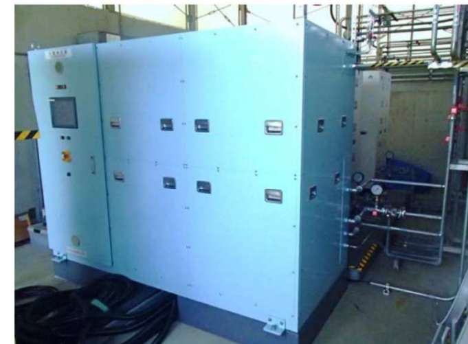
2015 Kyushu University PEM type WE for H 2 station(1Nm 3 /h)
